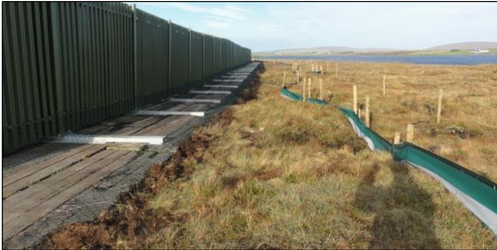
Plate 3-4 Silt Fence Details
