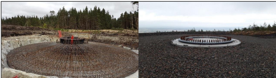
Plate 2-1 Turbine 'Anchor Cage' and finished turbine base
