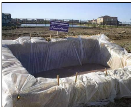
Plate 3-5 Typical concrete shoot wash out areas
