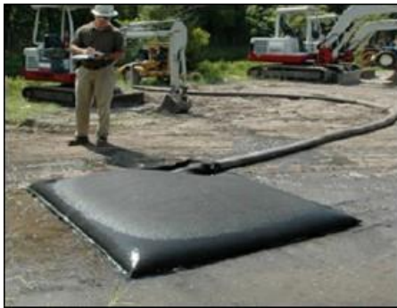
Plate 3-1 Silt Bag with water being pumped through
