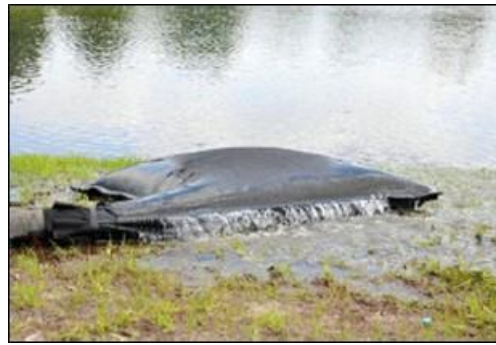
Plate 3-2 Silt bag under inspection
